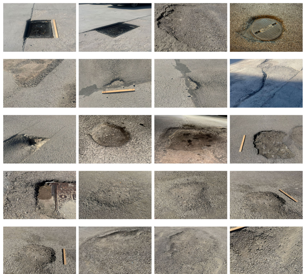
Figure 3. Field-collected images displaying isolated potholes captured in urban environments.
