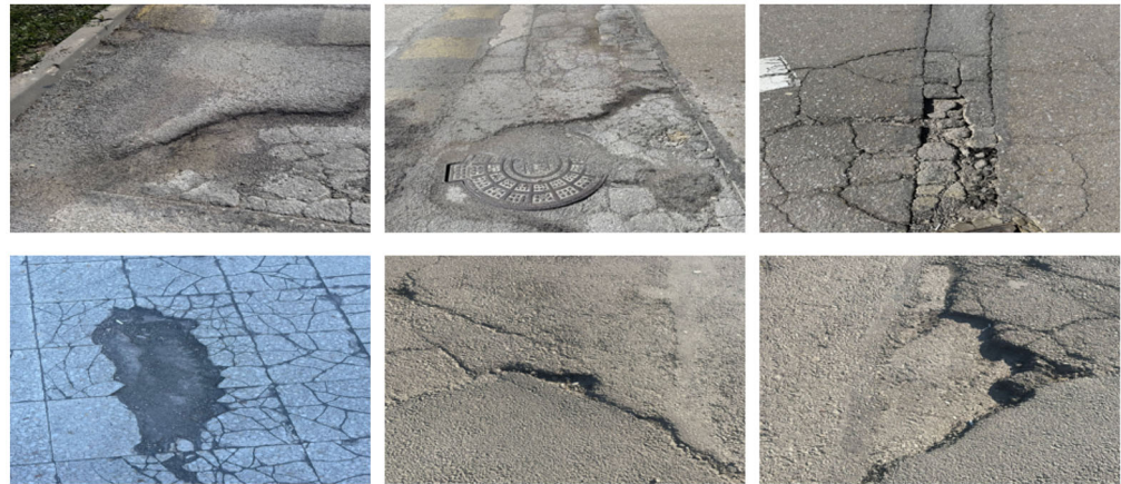
Figure 4. Field-collected images with combined road damages: coexisting potholes and cracks.
